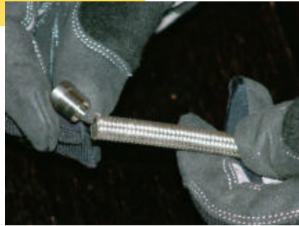
Place the ferrule at an angle to the hose. Make sure that the thin end of the ferrule goes on first.
